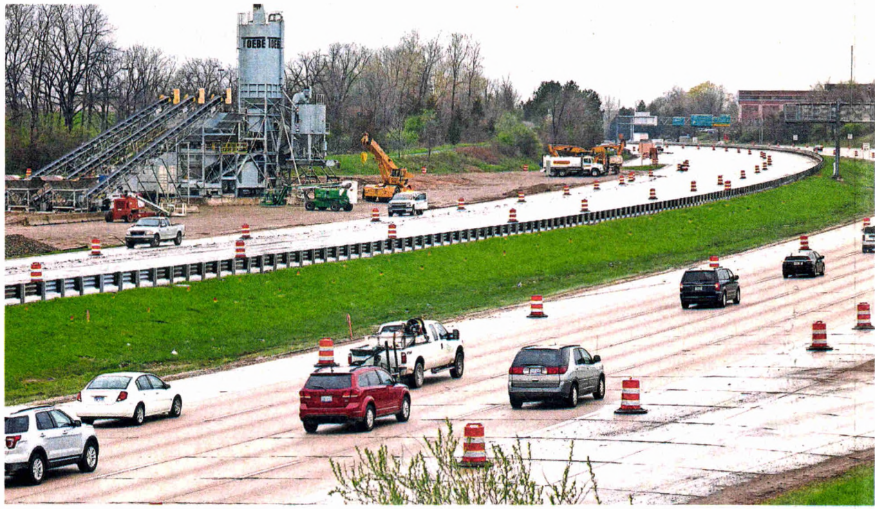
Northbound traffic was normal at mid-morning Monday. There was no southbound traffic other than construction-related vehicles. The concrete plant is up and ready.
