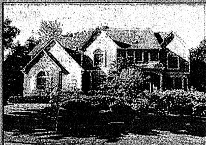
FARMINGTON HILLS $699,000 Over 5600 square feet. 2 Story Living room boasts Bay Windows overlooking the tiered Decking and yard backs to private woods and golf course. Finished Walkout. MLS 28117504 248-360-9100
