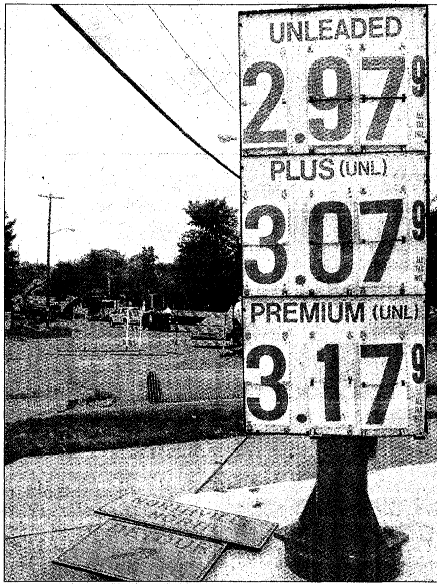
The Speedway station, located behind the barricades for the construction, is one of many businesses in Old Village affected by construction.
