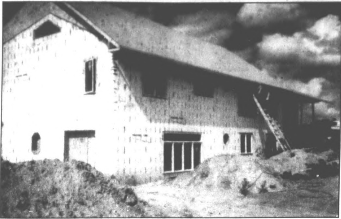
Concrete structure: This two-story house in Omaha, Neb., is being built with PolySteel insulated concrete forms. These forms, shaped like large egg cartons, are composed of polystyrene, an excellent insulator, and are reinforced by steel.
