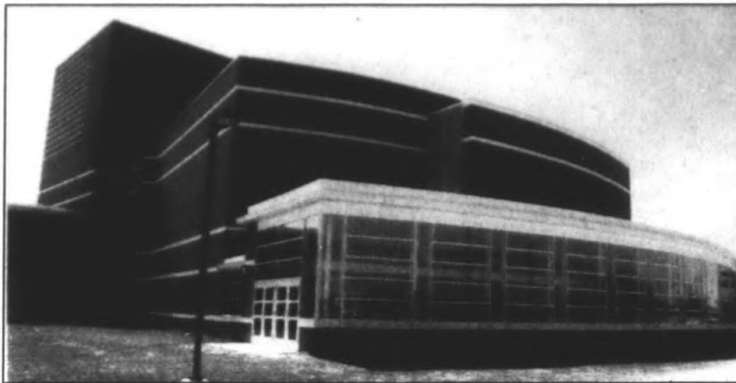
Kudos: The Troy High School design employs extensive use of glass and simple geometric shapes.
