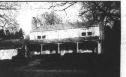
ANOTHER OPPORTUNITY To live in a 4 bedroom, 2 1/2 bath home designed by Clifford Wright and associates in downtown Plymouth. Updates include $9,000 in landscaping and brick sidewalks on a private lot 174 feet deep. Seller assisted financing is available. Asking only $269,900. REMERICA HOMETOWN REALTORS 453-0012
