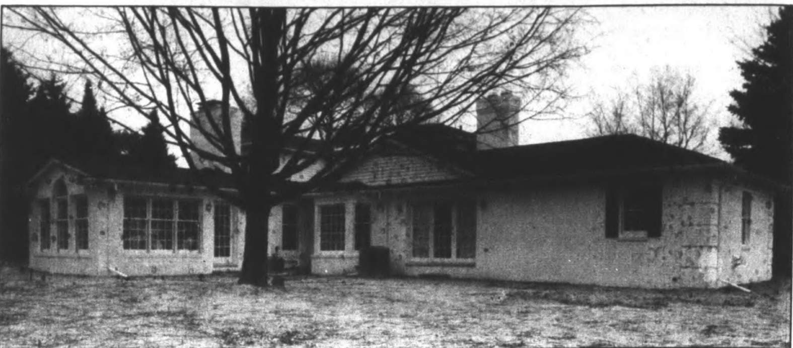
Living space boosted: This Bloomfield Village house, a two-story brick Georgian-style colonial, received an addition of 1,100 square feet to the original 3,100. The central entrance faces east (top). The additions were placed on the south and west sides of the house (bottom). A four-foot brick wall extension was placed on the south end of the second floor to expand the bedroom there. A master bedroom was added to the south end of the house, and a conservatory, with windows on three sides, was added to a family room on the west side, or back, of the house.
