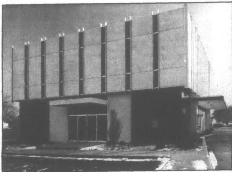
The old: a utilitarian structure.
