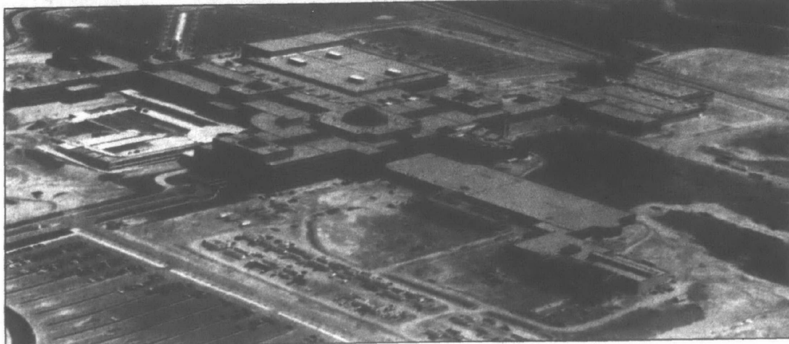
Central Energy Plant at Chrysler Technology Center.
