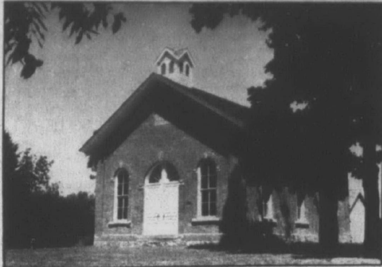
The school, at Plymouth Road and Gotfredson, was built in 1880 and used for many years until it closed in 1982.
