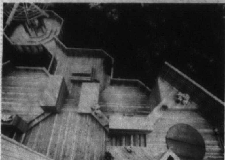
This multi-level deck in octagonal modules uses varying elevation levels, raised planters and screens to create privacy areas for a hot tub, picnic table and gazebo.
