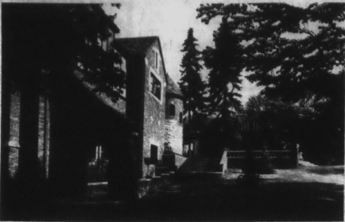
Materials used on the 4,500-square-foot addition to this house built in 1927 were the same as the original. Brick on the addition was hammered and chipped on site to match existing brick.
