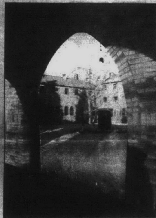
A view of the Cloister Garth. An old stone well lends Old World charm to this quiet garden retreat. The octagonal tower is pierced on all sides by graceful arches and topped by a weathervane bearing the Franciscan insignia.
