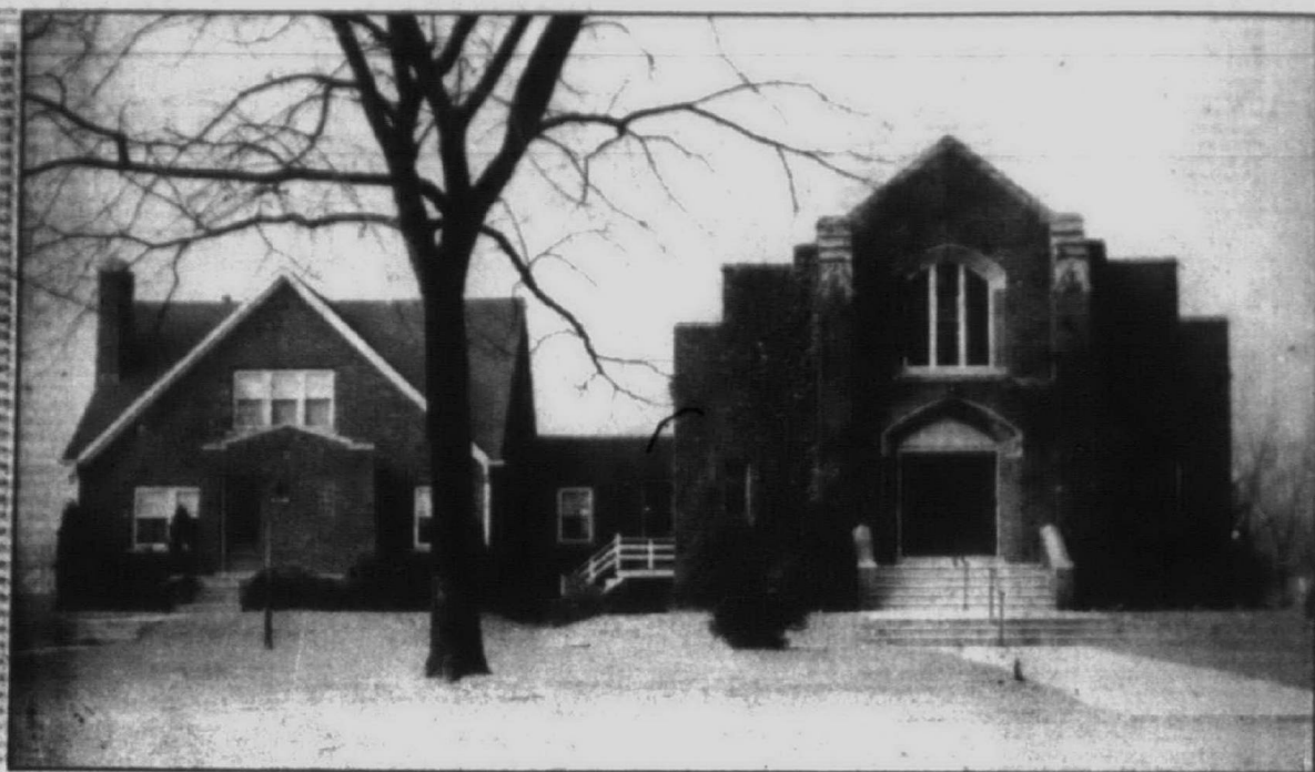
photo courtesy Garden City Presbyterian Church Garden City Presbyterian Church, built in 1928, has primarily an English Tudor influence, according to architect Betty-lee Seydler-Sweatt. Characteristic of the style is the Tudor arch, a low, wide arch that peaks above the church's wood doors.
