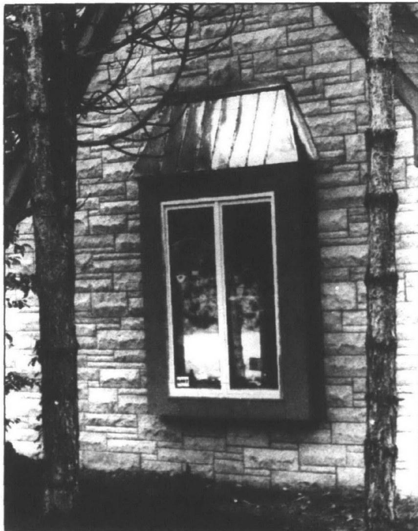
JOHN STORMZAND/staff photographer "Balmoral," Homearama Model 7, by Robert R. Jones Associates Inc., West Bloomfield, features an English colonial style with a European stone exterior.
