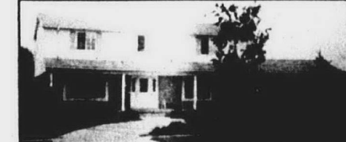
LOCATION PLUS CHARM. Plus value. 3 bedroom Plymouth condo. 2 1/2 baths, 1 car garage. Finished basement. For discriminating condo seekers. Located in a well maintained complex and park like setting. $135,900 455-7000
