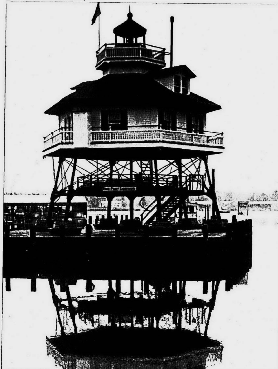
The Drum Point Lighthouse in Solomons, Md., makes a picturesque reflection in the water. — photos by MICKY JONES
