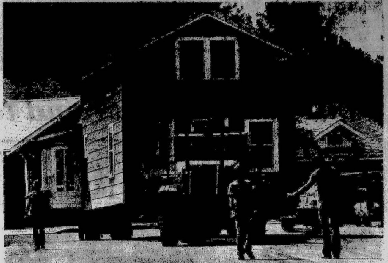
The gray house, now on wheels, moves slowly down Starkweather toward its new location.
