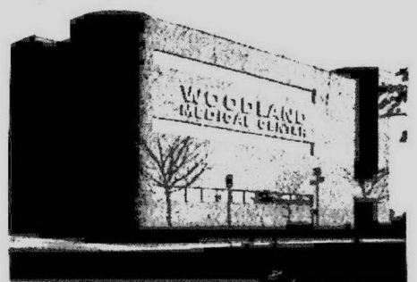
Woodland - Novi 41935 W. 12 Mile Rd., Novi, Michigan
