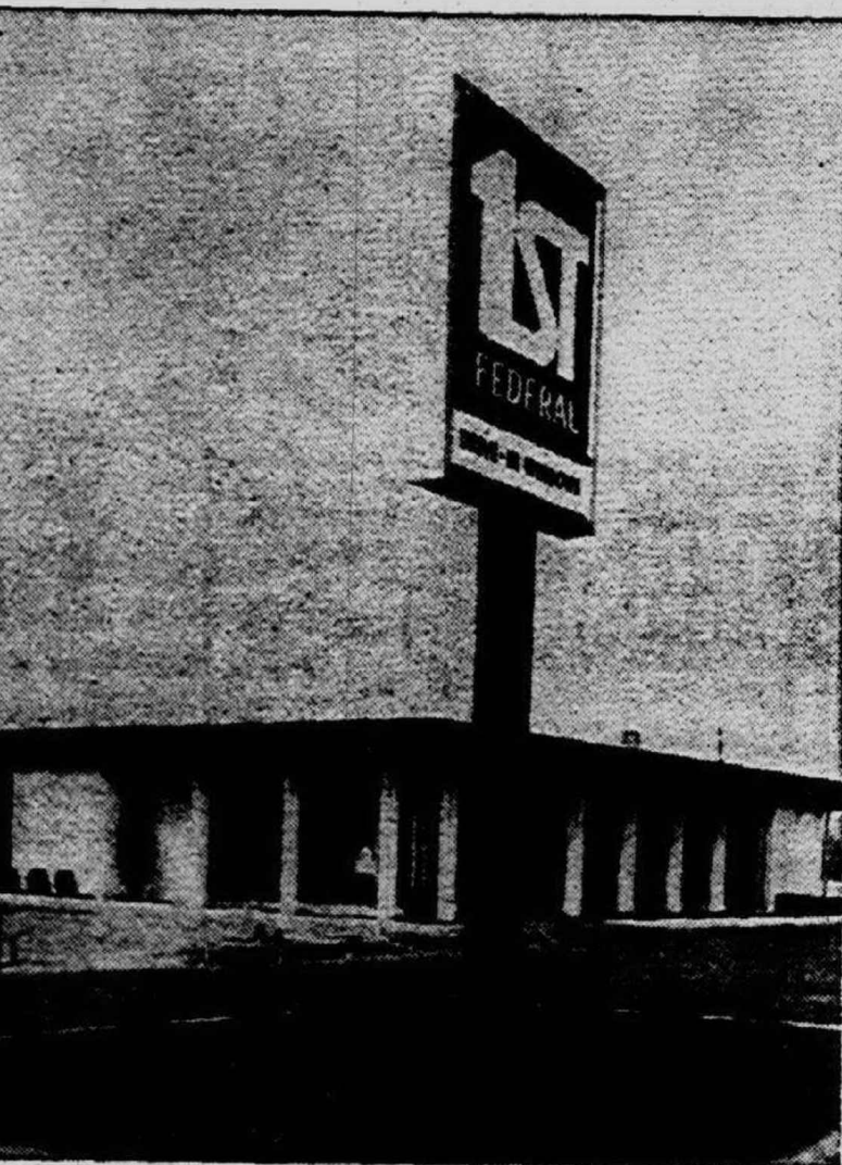
NEW MODERN BRANCH of First Federal Savings and Loan Association will hold a grand opening Friday. The new structure is located near the intersection of Middlebelt and Seven Mile Roads, across from the Livonia Mall.
