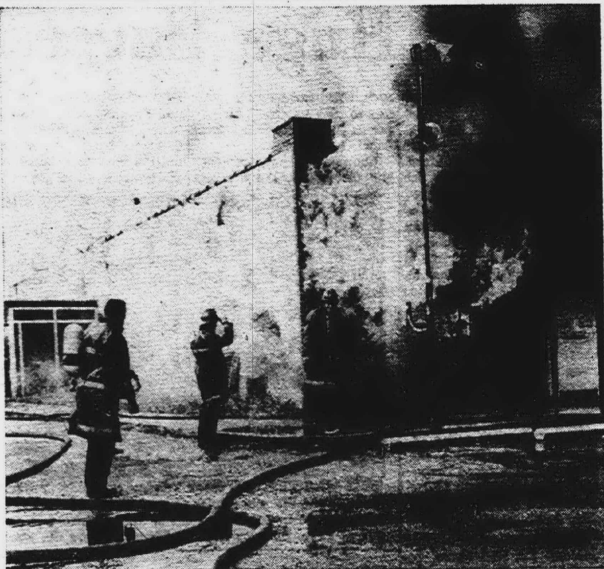
FLAMES, SMOKE engulf Livonia firemen as they battle the fiery blaze that completely gutted Pandora's on Plymouth Road. The fire broke out shortly before noon and even though the fire department rushed all available equipment, the interior was destroyed before the flames were extinguished.
