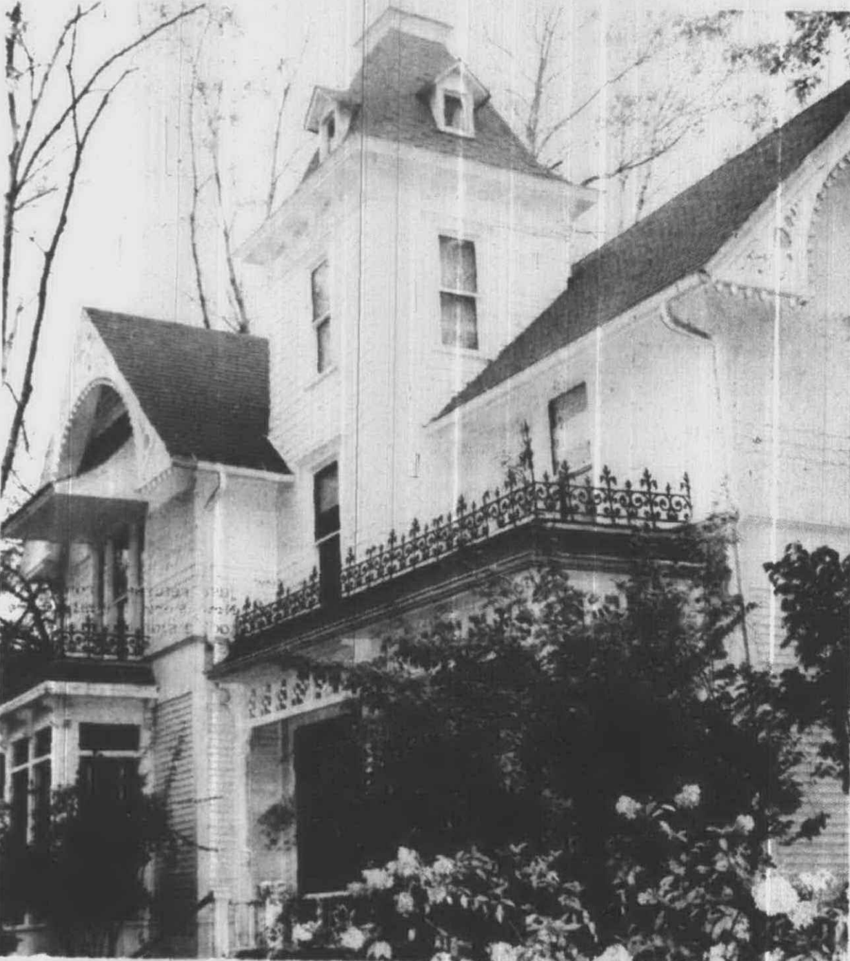
This view of the house shows the broken facade and elaborate wrought iron work rarely seen any more.
