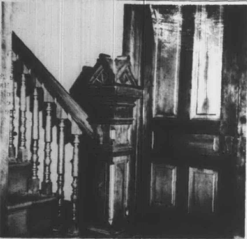
The elaborate newel post is made of walnut. The doors behind are the old sliding doors that were used to separate rooms.
