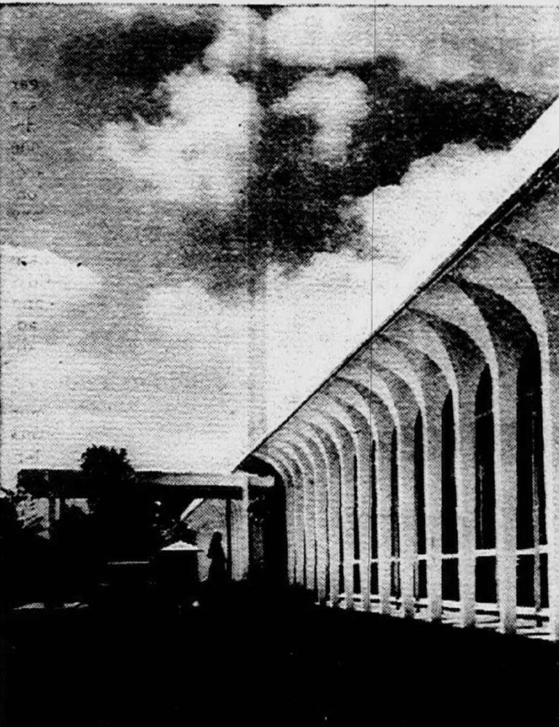
ENTRANCE TO PROVINCIALATE — White concrete colonnades capture both majesty and simplicity along vincialate. Motif is repeated along front of Mother of Mercy Novitiate.
