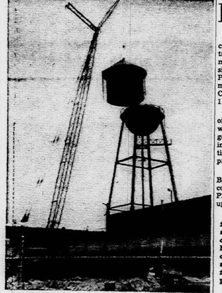
**ANOTHER PLYMOUTH landmark faded out of existence** last week when workmen razed the water tower at the old Continental Can plant on Junction. Jim Allison is riding the crane as the top is lifted from the tank. The work was handled by the Plymouth Excavating Co., headed by Tom Clinansmith.
