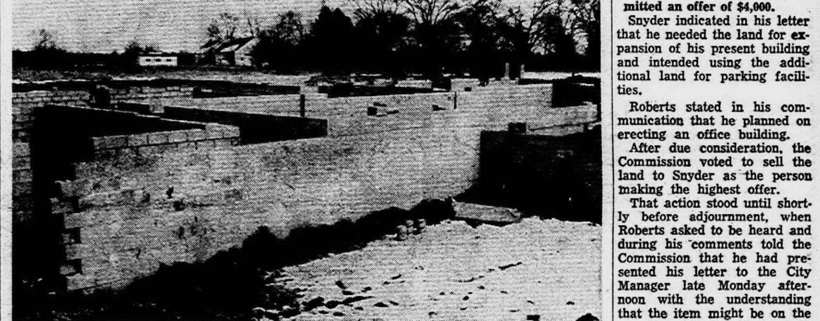
BUILDINGS LIKE THIS are big reasons for the need for industrial and commercial expansion in the Plymouth Community. This shows the work on the new elementary school on Five Mile Road near Schoolcraft, which has a target date of September, 1967.
