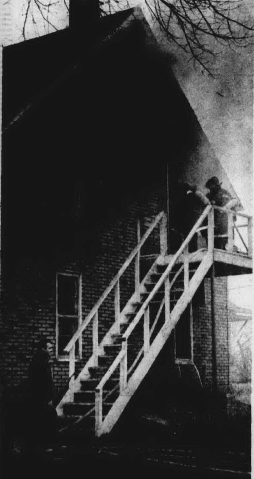
CHILDREN PLAYING with matches caused a fire which swept through the inside of this home at 289 Pearl St. Saturday around noon. City firemen report the fire had gone too far for them to stop extensive damage to the interior of the two-family home.
