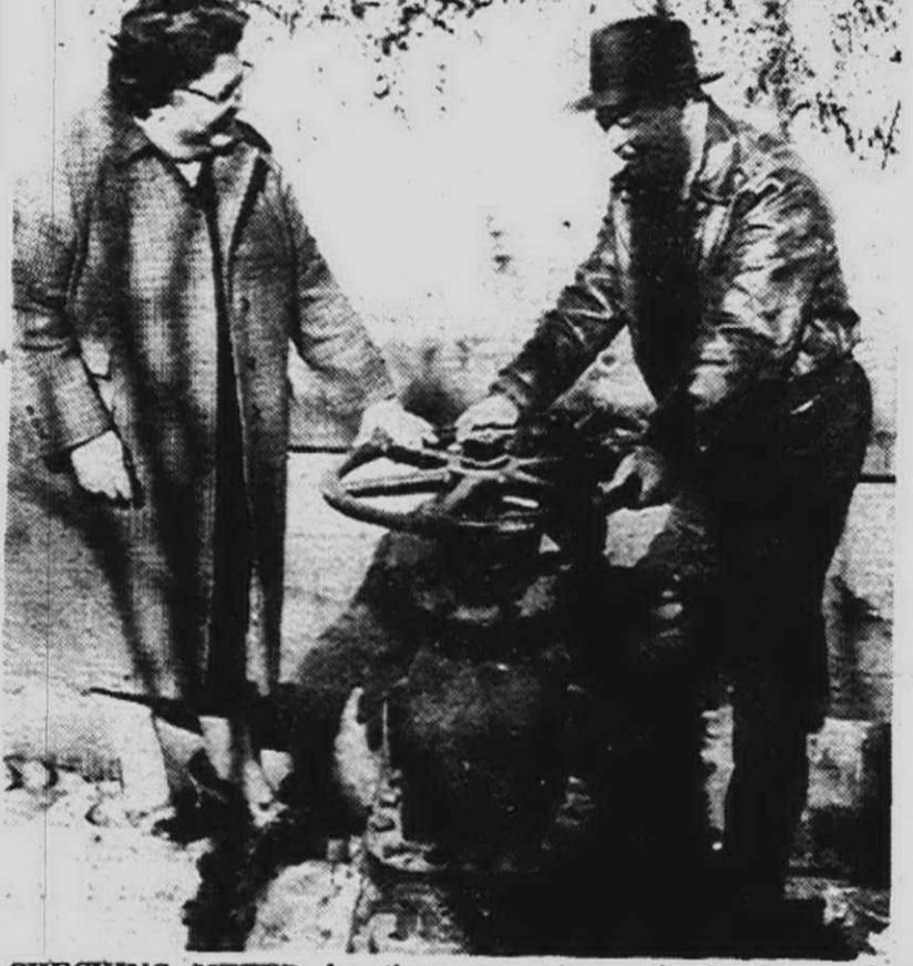
CHECKING METER for the new water main to Plymouth Township are: Township Clerk Mrs. Elizabeth Holmes, head of the Township Water Department, and Engineer Herald Hamill. The new line will furnish water to the west side of the Township and figures to open that area for the greatest development in Township history.
