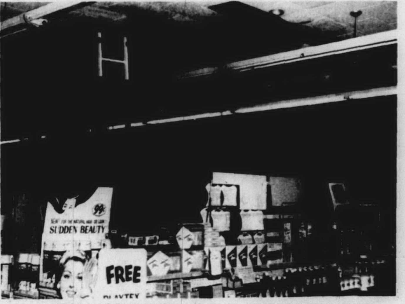
FIRE IN THE CEILING at Consumer's Discount Store on Forest Ave. downtown sent mid-day shoppers scurrying Tuesday afternoon. An overheated light fixture was figured to have caused the blaze, which was stopped in record fast time by City firemen. Smoke and water damage was comparatively light; fire damage was confined to a small area of the ceiling.
