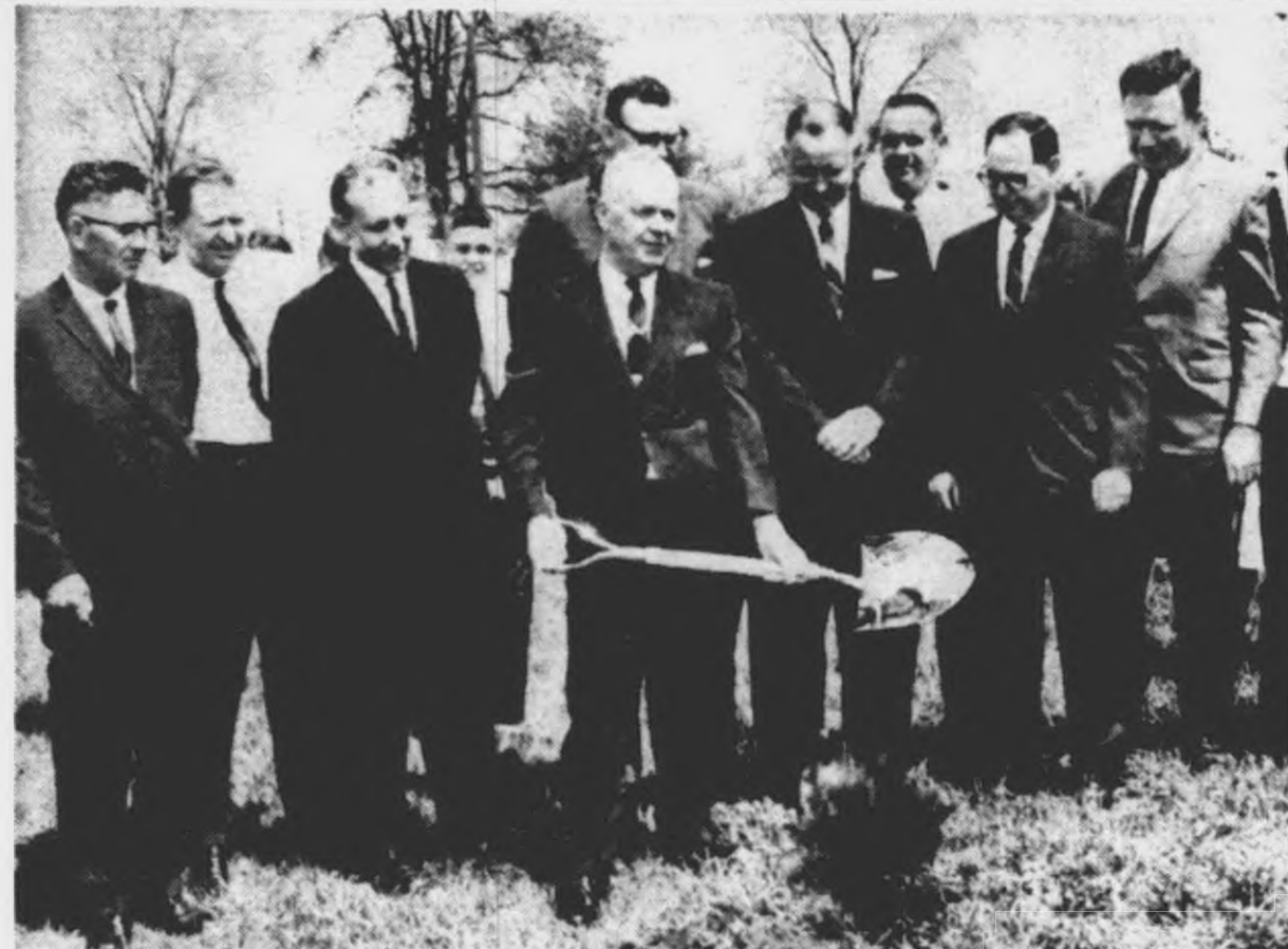
BREAKING GROUND for the new $400,000 church and educational unit of Calvary Baptist Church is Rev. P. J. Clifford, who is shown turning the first shovelfull of dirt. The new church will be erected on a 9½ acre site at 43065 Joy Road in Plymouth. Members of the Building Committee watch Rev. Clifford and
