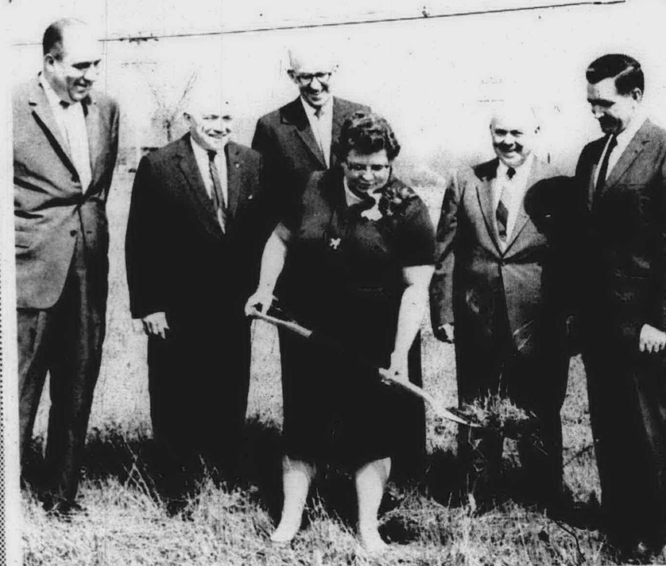
MICHIGAN NATIONAL BANK broke ground for its new building on the corner of Sheldon and Ann Arbor Roads last Thursday, and Township officials were on hand to help. The bank will be a colonial type structure, and will replace the trailer currently serving as the bank's outlet. Jeff Reaume, John McEwen, Township Supervisor, Joe Salisbury, C. V. Sparks, Township Clerk and Edwin Jones look on as Township treasurer Elizabeth Holmes breaks the ground.
