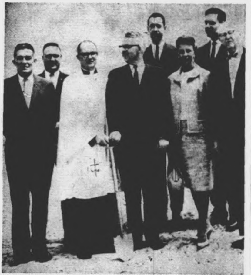
GROUND WAS BROKEN recently for the first unit of the Lutheran Church of the Incarnation building on West Ten Mile Rd. in Farmington. Participating in the ceremonies were from left: front row, Kenneth Maahs, Rev. Robert Zoeller, Robert Eckel, Mrs. John Weightman and William Kleuscher; back row, Richard Brewington, Raymond Fitzsimons and George Poertner.
