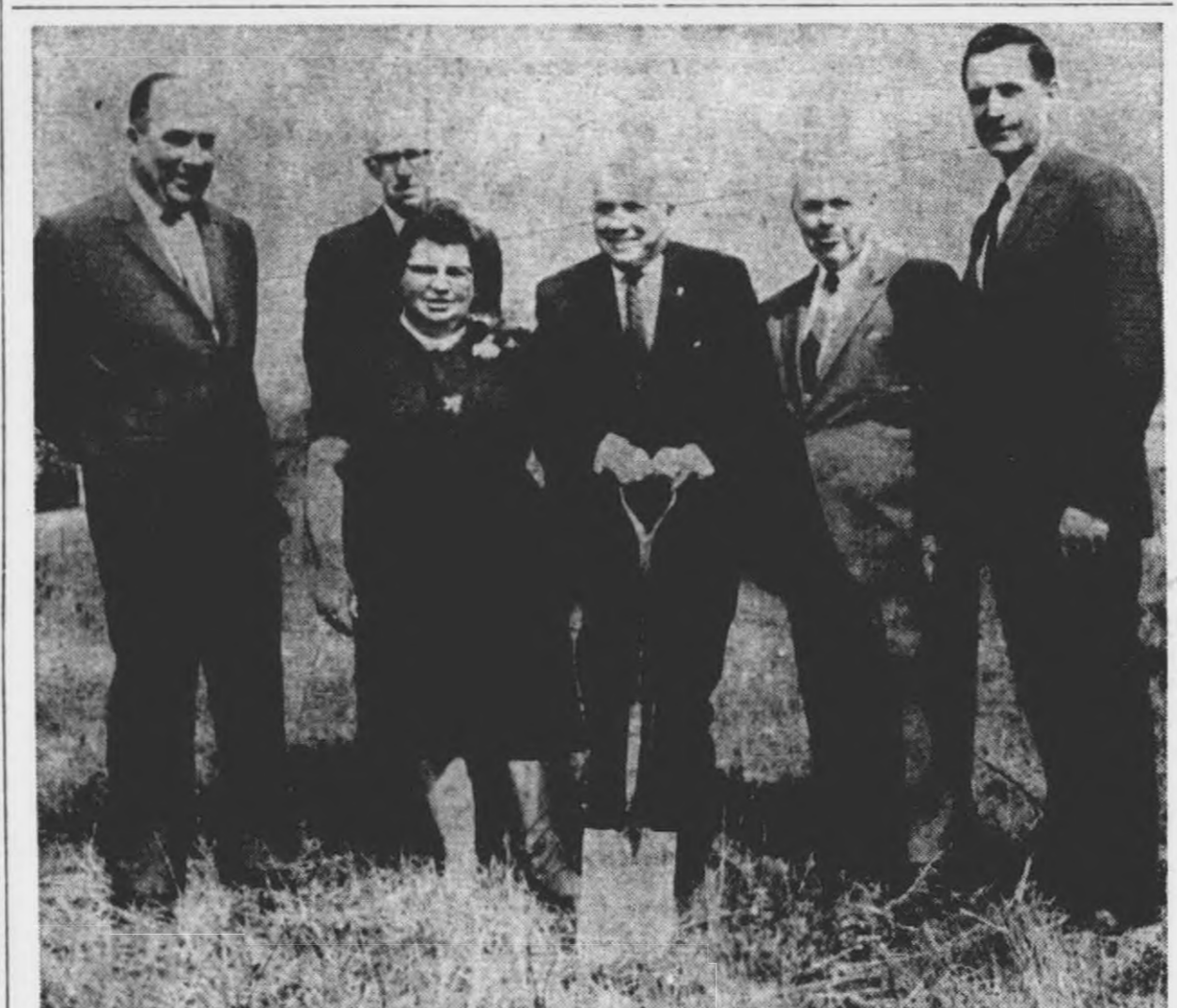
BREAKING GROUND for the new Michigan Bank branch building at the intersection of Ann Arbor and Sheldon Roads, is Plymouth Township Supervisor Sheldon McEwen. Bank officials have a target date of 3 months for construction and opening of the branch which is now quartered in a trailer. Participating in the ceremonies were: (from left in front) Township Treasurer Mrs. Elizabeth Holmes, McEwen and Township Clerk C. Veach Sparks, (rear from left) Branch Manager Eugene Reaume, Vice President Joseph Solsbury and Vice President Edwin Jones.
