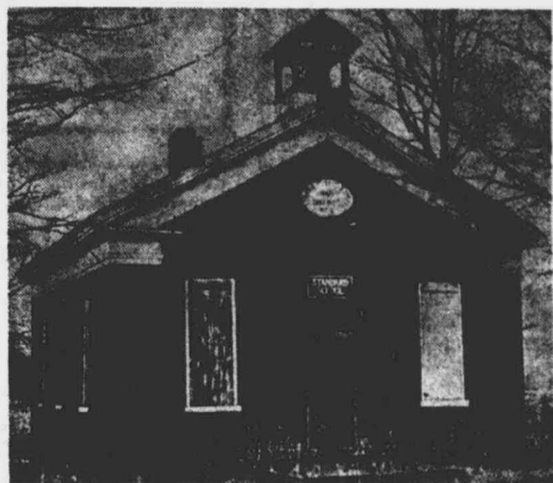
STANDARD SCHOOL, one of the first "little red schoolhouses" to be built in Michigan has stood for many years on Six Mile and Newburgh Roads.
