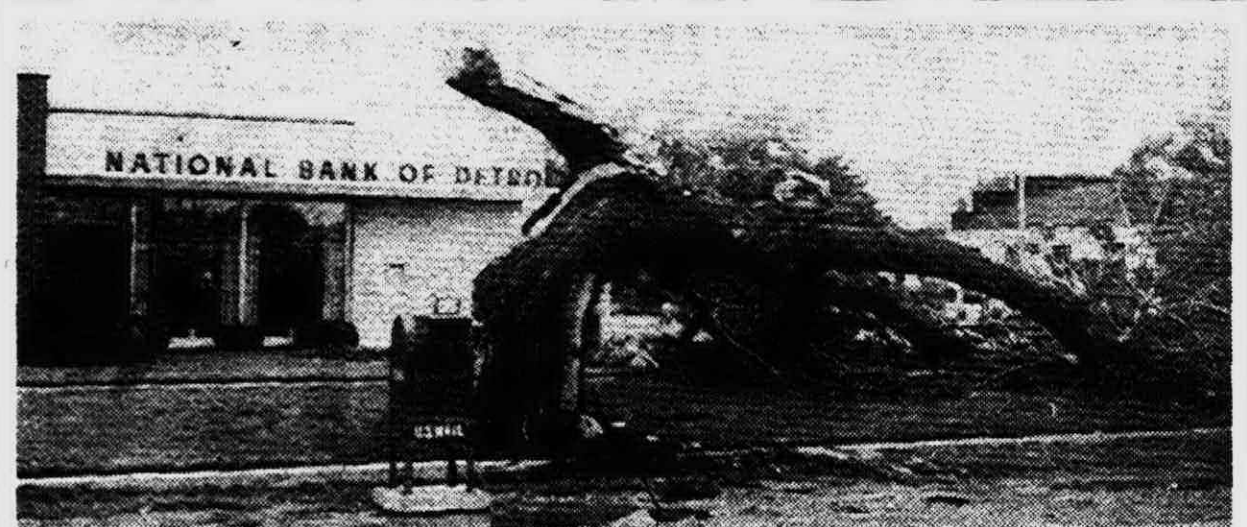
FRIDAY'S STORM uprooted this big tree in front of the National Bank of Detroit's branch on Ann Arbor Road in Plymouth. The tree fell towards the bank but was still some 25 feet short of hitting the building.
