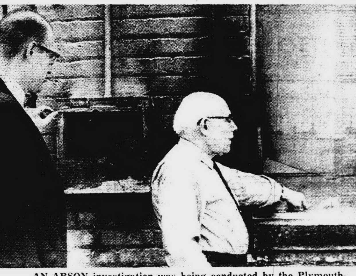
AN ARSON investigation was being conducted by the Plymouth Fire Department this week following two fires behind stores located adjacent to the City's Central-Parking Lot. Hugh Jarvis, of Hugh Jarvis Gifts, left, and Isadore E. Kades inspect a shattered plate glass window and a damaged meter box behind Kades Store at 868 W. Ann Arbor Tr.
