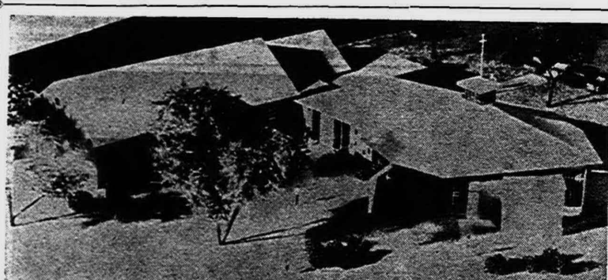
TRINITY CHURCH of the Brethren, when a new building program is completed, will soon take on this appearance.
