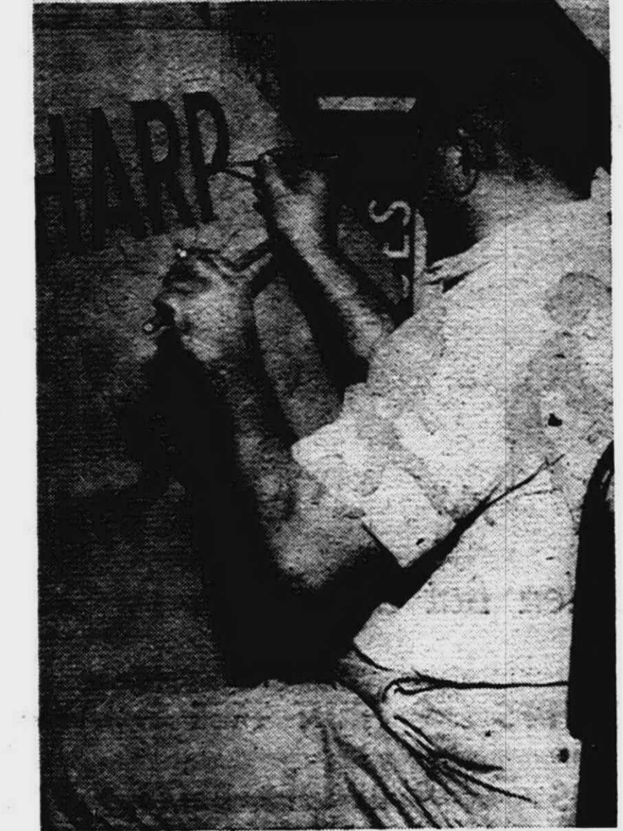
ORDERS for one or two signs of a kind are hand painted at the shop. Here, painter Jerome Yelinek of Livonia hand letters a sign. Yelinek said he can finish a sign with 6-inch letters in about 15 minutes.
