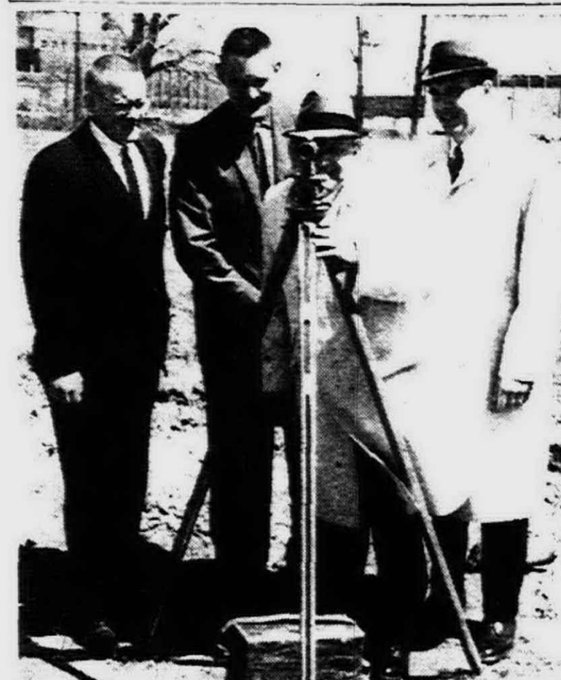
GETTING A LINE on the site of the new Thermax Co. building in Plymouth's Industrial Park are: (from left) Chief Engineer Reuben Aho, Plymouth City Commissioner George Lawton, Ben Milt, president and general manager of Thermax; and Plant Manager Earl Opliger. Work has already started and Milt hopes to be in the new plant within 90 days.
