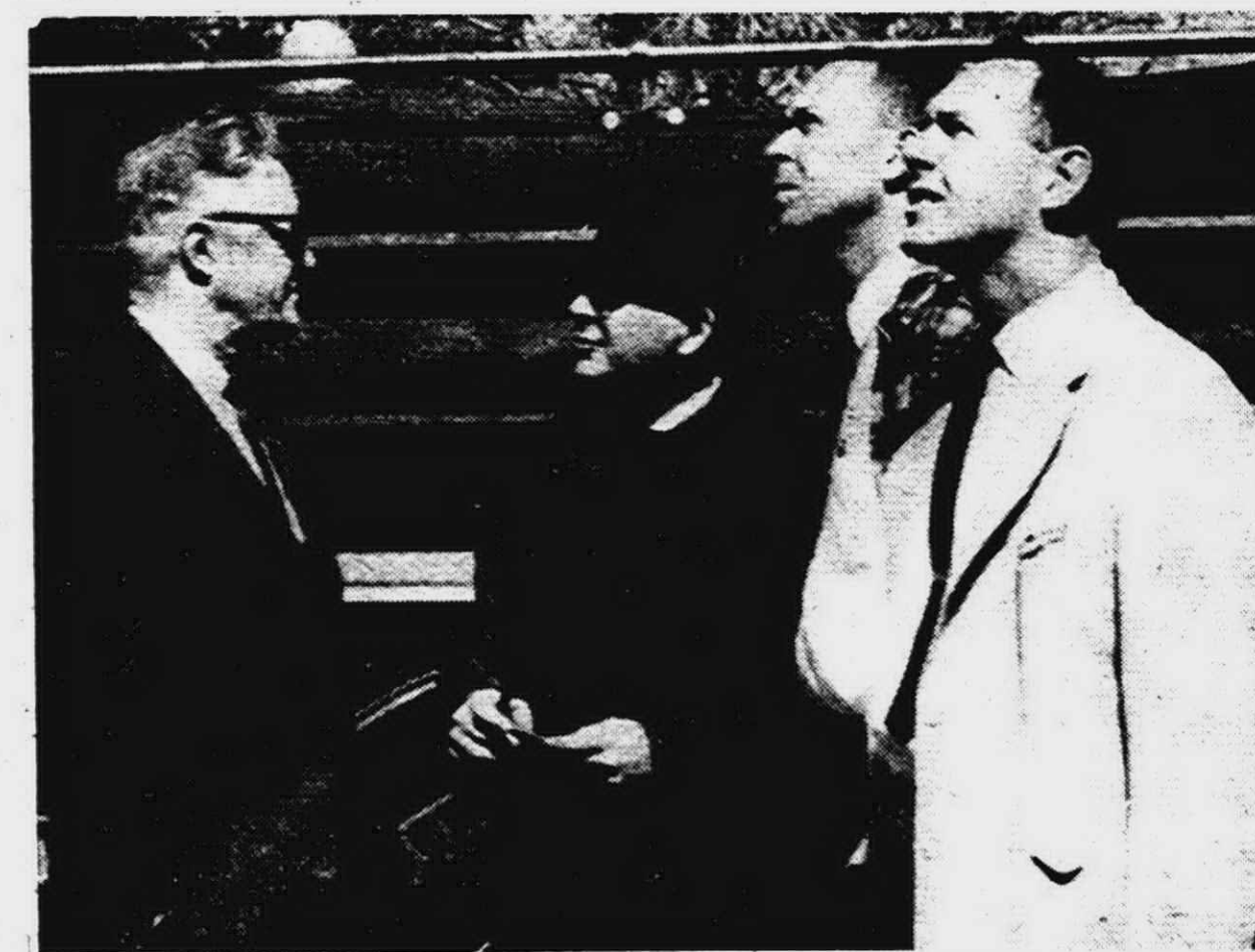
PRESIDENT of Distribution Services, Inc., W. C. Scott, left, talks to local restaurateur Robert Stremich, and sons, Phil and John Scott, as they watch the dismantling operation at the old Daisy plant.
