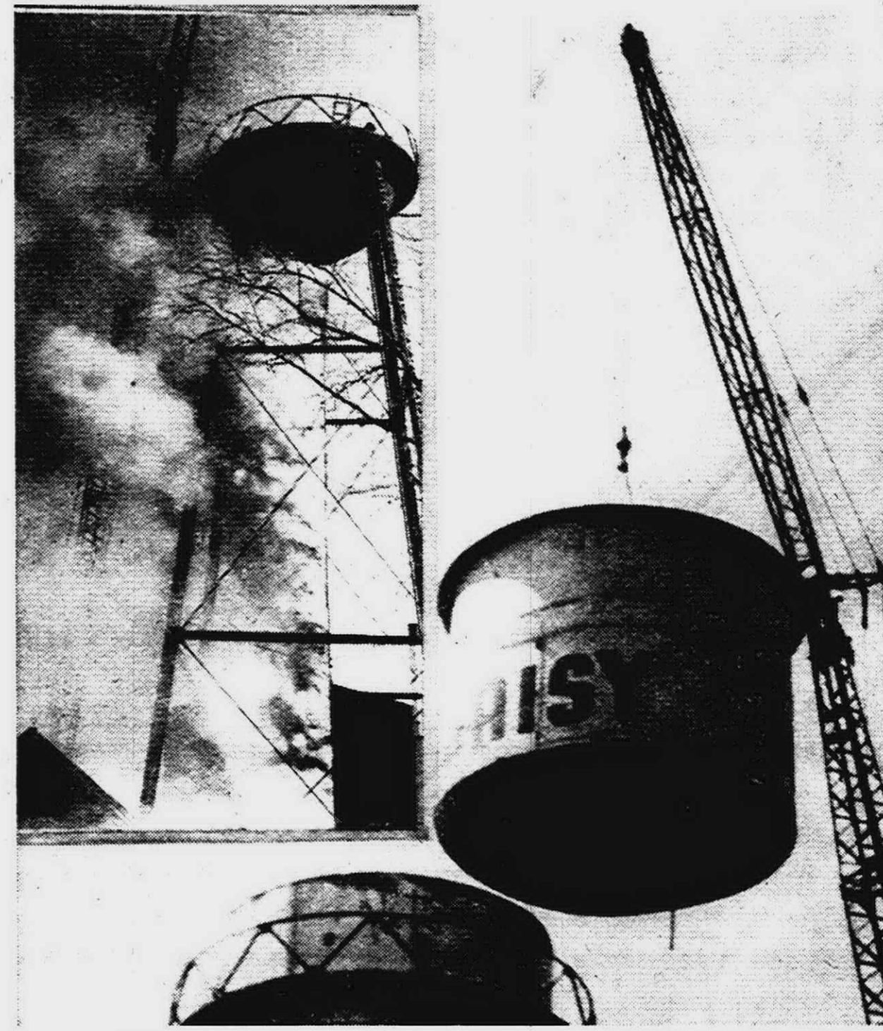
TWO MAJOR landmarks in the City of Plymouth were removed from the local scene last week as workmen dismantled both the old Daisy water tower, located at the Distribution Services, Inc. plant, and the black water tower located next to the former King Plant. Above, right, a huge crane lifts the top off the Daisy tower after a workman had cut it away with an acetylene torch. Left, the wood-covered center pipe caught fire Wednesday as sparks from a workman's torch ignited it as he worked to dismantle the King tower. Plymouth firemen were on standby status Tuesday and Wednesday at both sites.
