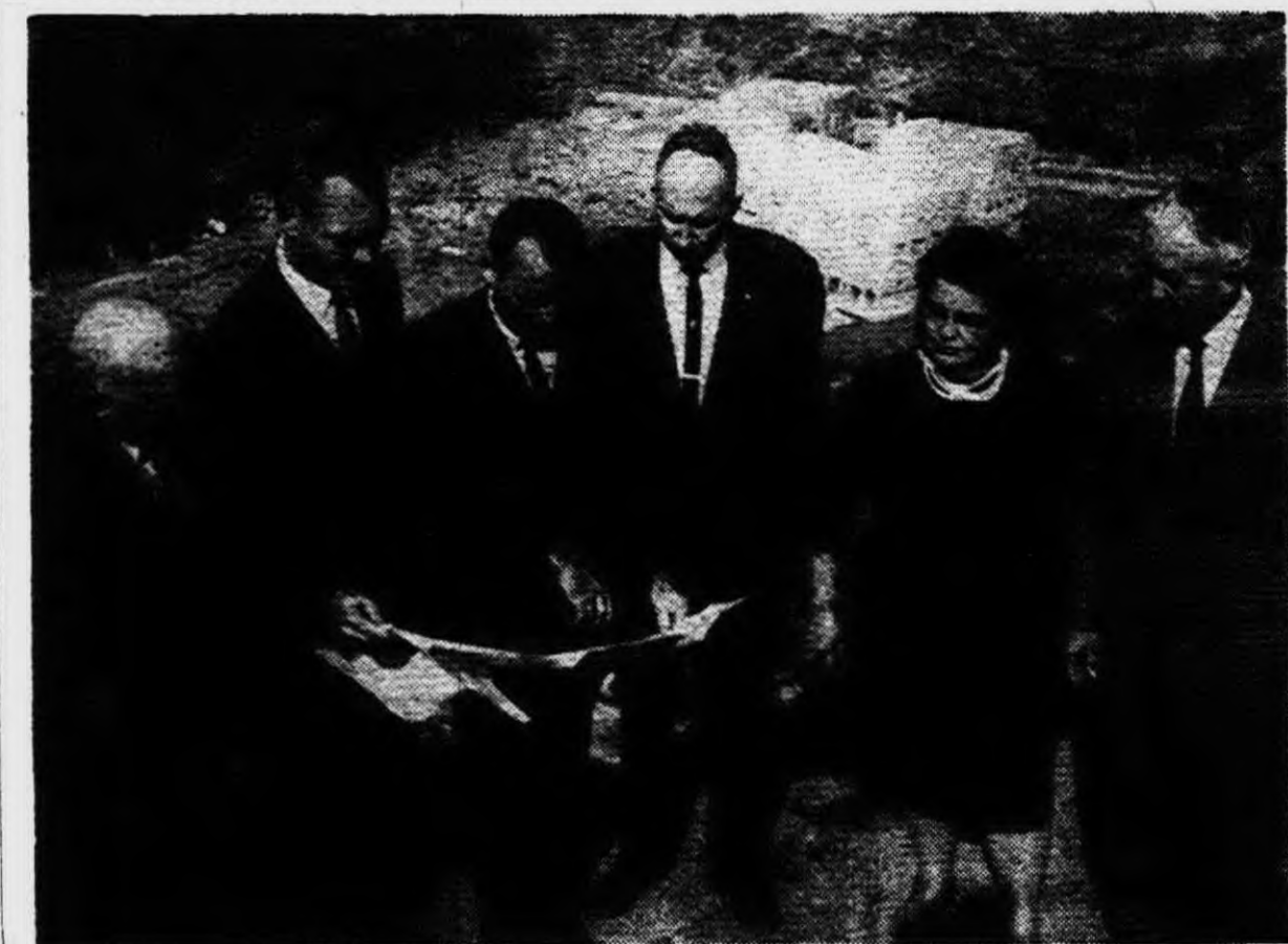
STUDYING PLANS for the new Professional Building under construction on Sheldon Road, north of Bird School, are: Plymouth Township Clerk John McEwen, Dr. David McCubrey, Builder Loren Gould, Dr. Walter Hammond, Township Treasurer Mrs. Elizabeth Holmes and Township Supervisor Roy Lindsay. Gould hopes to have the building ready for use within four months and expects to have eight doctor tenants. Dr. McCubrey and Dr. Hammond are the first to sign contracts. The footings are in as the picture shows, and workmen will begin the building shortly.
