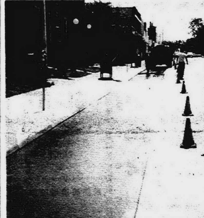
RESURFACING of Penniman Ave. kept workers in Plymouth's Department of Public Works on the go last week. They are shown completing a strip in front of the Post Office building.
