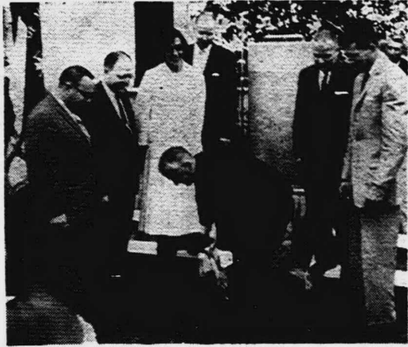
DIGGING FIRST SHOVELFUL of dirt is Schoolcraft College Board Chairman Harold Fischer, of Plymouth, at the groundbreaking ceremonies Saturday at the campus site at the intersection of Haggerty and Seven Mile Roads. Surrounding Fischer are members of the Board including (from left) Paul Mutnick, Clarenceville; Clarke Oldenburr, Garden City; Mrs. Jane Moehle, Plymouth; James O'Neil, Livonia; Erwin Brown, Livonia; and Charles Kirkpatrick, Livonia.
