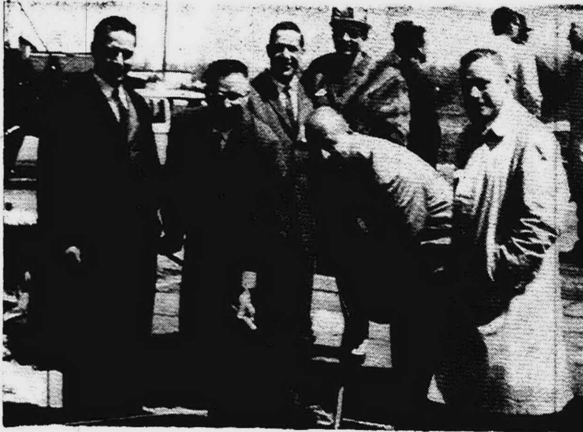
FIRST SHOVEL of dirt for the new Angelo DiPoni Co. building is lifted by Mayor Harvey Moelke along with President Angelo DiPonio at the official ground breaking ceremonies.
