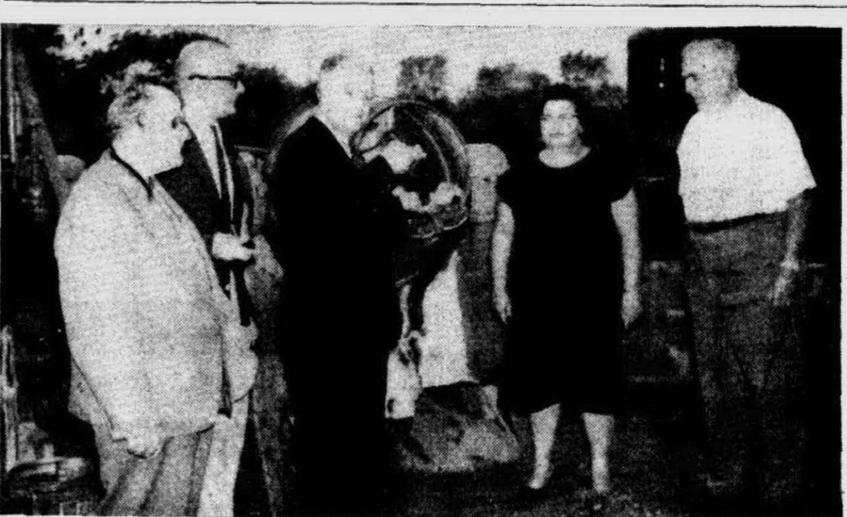
GROUND BREAKING ceremonies for the new $26,000 Department of Public Works building were held in Plymouth Township Saturday. Giving the contractors, who have the building well underway, a lift by shoveling gravel into a cement mixer was Township Supervisor Roy Lindsay. Looking on are Township Trustee C. V. Sparks, architect Tivadore Balogh, Township Treasurer Elizabeth Holmes and Township Trustee Louis Norman.
