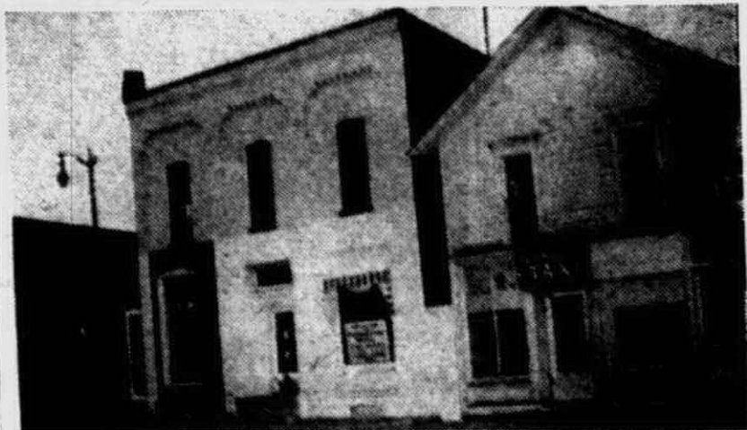
COMING DOWN SOON will be one of Plymouth's old blocks of stores. The buildings will be razed to make room for a possible municipal parking lot for temporary use until new tenants are found for the land. Clearance will begin next month.
