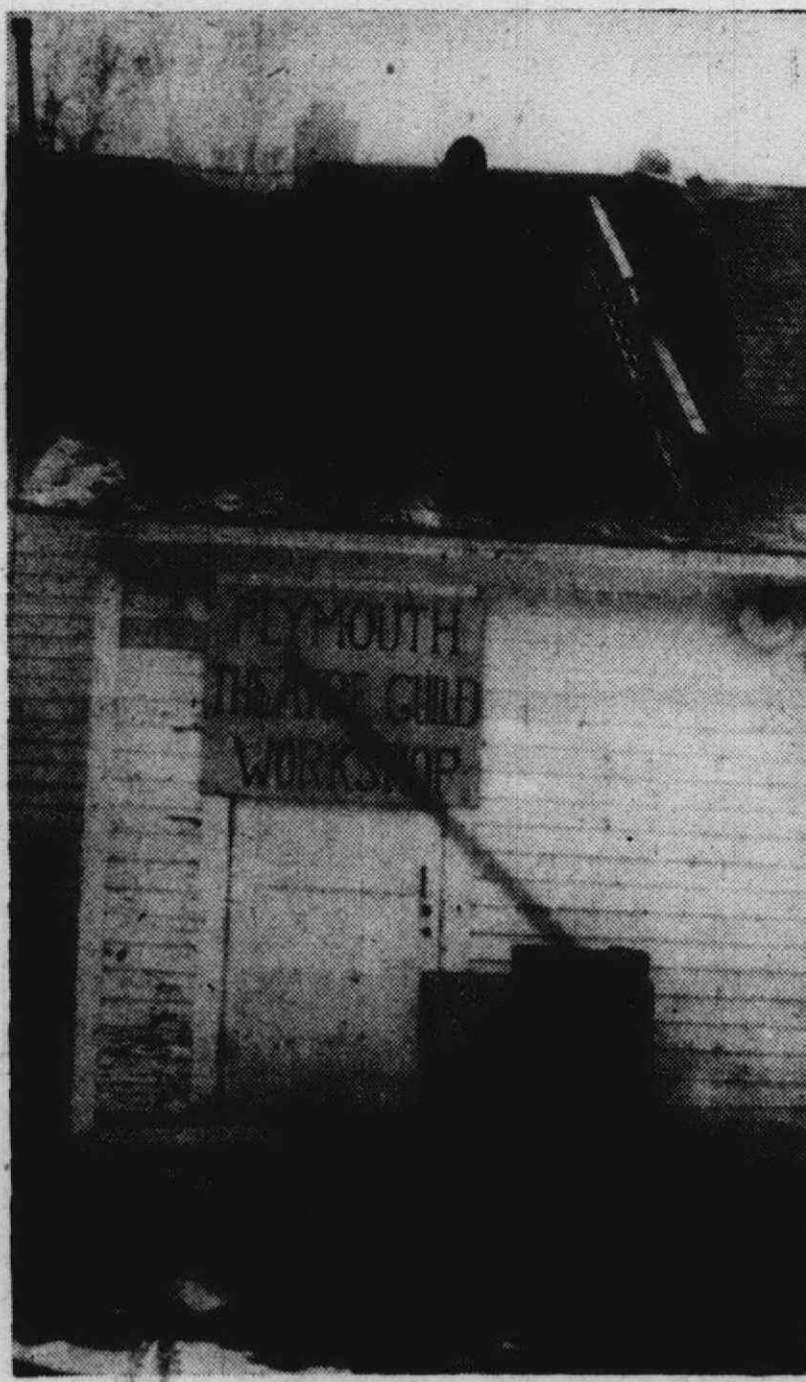
CLOSED AT least for a while will be the Plymouth Theatre Guild Workshop at Bartlett School. Fire starting from a furnace crept through the roof and nearly all of the contents suffered some type of damage. Story on front page.
