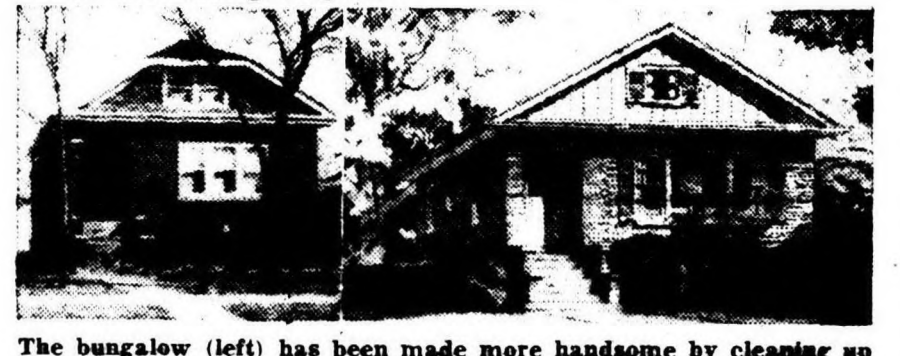
The bungalow (left) has been made more handsome by cleaning up the roof lines and adding more modern windows.
