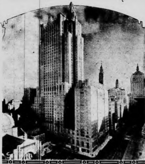
This hotel, said to be the tallest in the world, has just been opened in New York. It is the new Waldorf-Astoria. The view of it is taken looking south on Park avenue.
