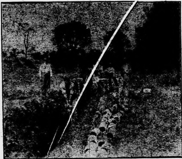
Agricultural Students at Michigan Agricultural College Constructing the Drain.
