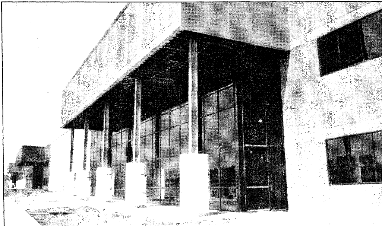
Big, eh? Well there's more on the way. Ashley Capital's confidence in P-C-N's commercial real estate market was strong enough to build not only this 450,000-sq. ft. multi-tenant facility on spec (without first having a buyer), but to begin further development at the 230-acre site on Michigan Avenue and Beck Road. Bay Logistics has moved into 110,000-sq. ft. of this building. (Crier photo by R. Alwood, Jr.)
