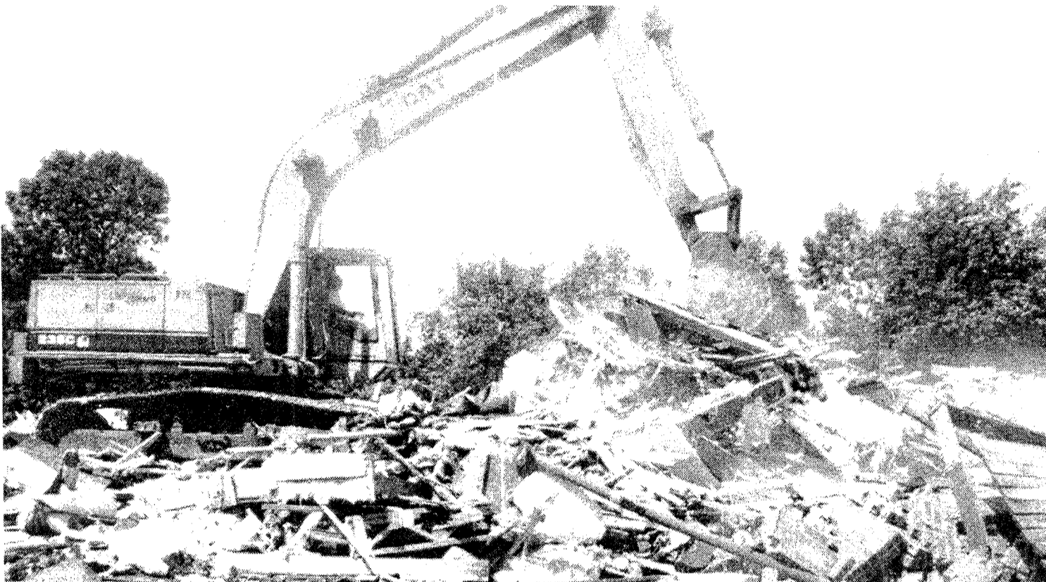
As bulldozers tear down three buildings at Plymouth Square Apartments to make way for a new Kroger grocery store, community officials should take heed: this may be the future of development in Plymouth-Canton-Northville. (Crier photo by Scott Goodwin.)
