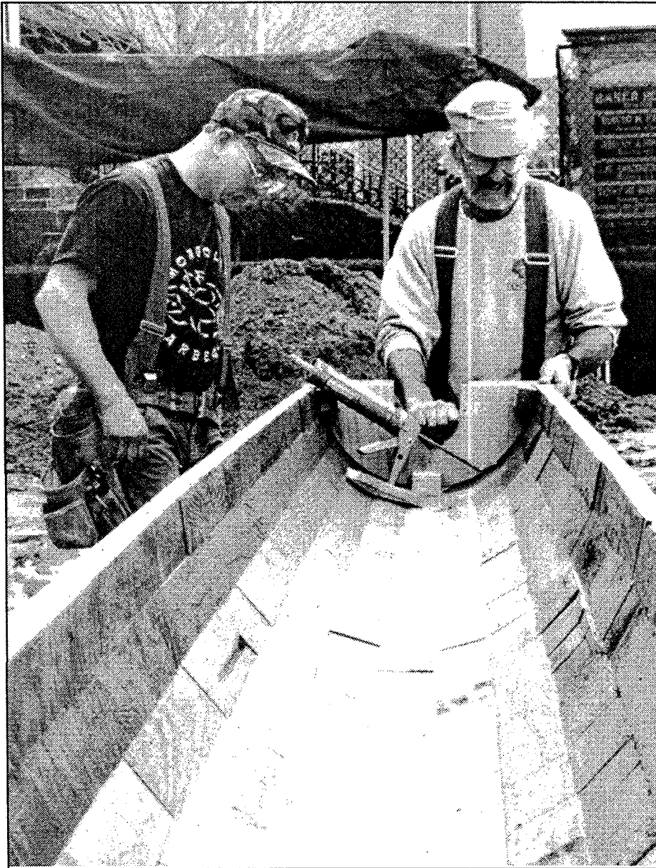
Ron Mazurek and Jim West (above) glue the bottom on to one half of a column shell that will grace the front of the new library. Made of water-proofed redwood and topped with a ceramic Erechtheum capital with necking, the columns will maintain the neo-classical theme set by neighboring City Hall and the Plymouth Historical Museum. Mazurek's and West's employer, Trendmill Works, did all of the library's finished woodwork. Inside, Joe Costa from Palmer Installations (at left) looks closely at a floorplan that shows which areas get which type of the more than 5,000 yds. of carpeting being laid.
