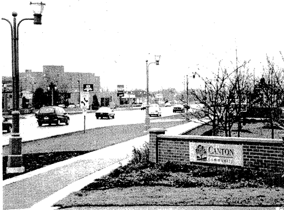
Elements of Canton's Downtown Streetscape, including streetlights and brick walls will be a part of the landscapng requirements for every new business being developed in the Downtown Development District. The requirements also holds true for existing business doing extensive remodeling, but not to new stores in strip malls. (Crier photo by Jessica McCartney).
