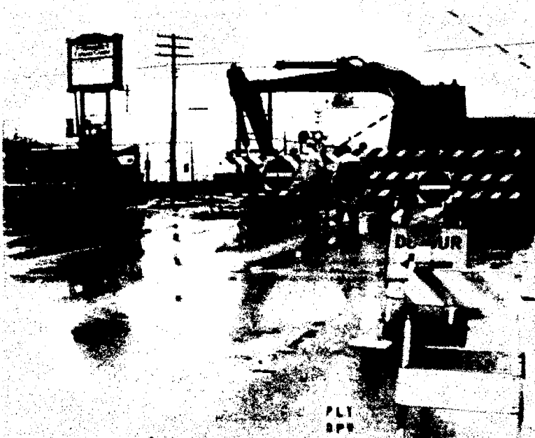
Work continues on the Main Street railroad crossing. Traffic has been detoured along Theodore and Farmer the last two weeks. (Crier photo by Tim Shuller)
